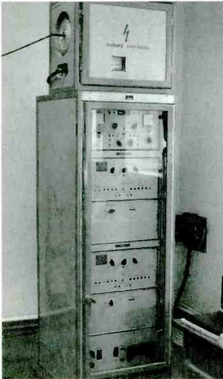
approximately 7000 meters from the end of the runway, with a 1000 W or 400 W/1020 Hz tone. One or the other NDB pair is turned on/off from the Air Traffic Control Tower, depending upon wind direction.
