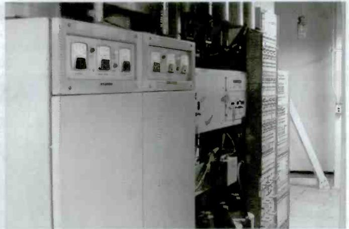
*Located on the lower level of the control center is the IRCS equipment. In the foreground are two General Electric transmitters (one active and one standby). In the middle is the antenna coupling system with more than a dozen large cavity filters, and in the background are all the receivers, demodulators, selective call tone generators, and other diversity gear.*
