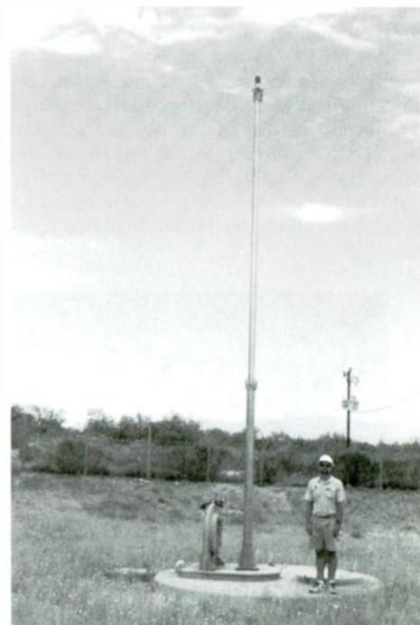
*The telescoping HF antenna is kept in its own hardened silo. It can telescope to as high as 117 feet depending on the frequency in use.*
