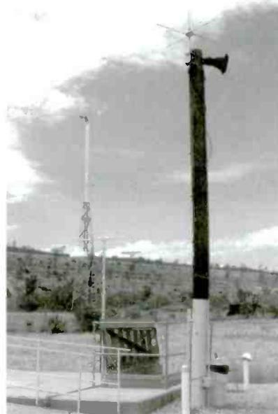
*The VHF RTMN antenna is mounted on a pole near the access portal. In the background is the main IRCS frequency diversity antenna.*
