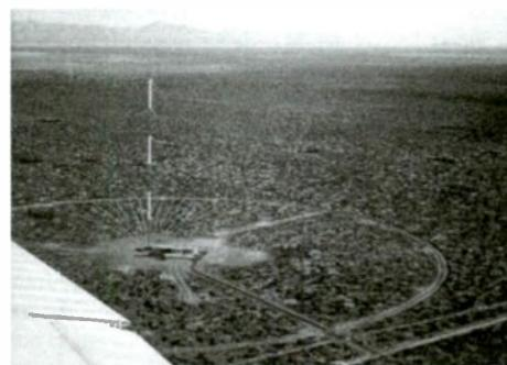
A typical LORAN transmitter
