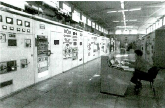
*Krasnyy Bor near St. Petersburg: a typical Russian transmitter hall with high power equipment from Komintern. The site has one 1000 and three 2000 kW LW/MW transmitters, as well as eighteen 200 kW SW transmitters that can be used in pairs.*
