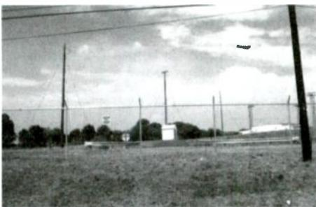
Figure 1. NXX/388 kHz, Willow Grove, PA – Transmitter is housed in the small shed; antenna wire is strung between the utility poles.
