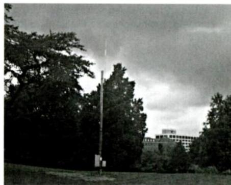
*The self contained 10 watt AM radio station KFQ-70 has a typical range of 4-6 miles. Tower height is 49 feet. Photo, courtesy NIH.*
