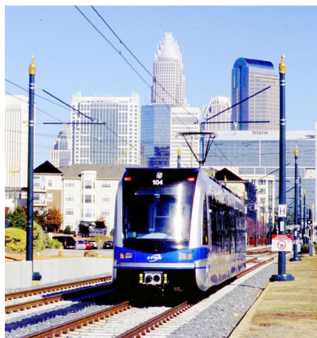
Charlotte, NC's Lynx light rail system is one of the newest in the country, having opened in November of 2007. Here a single-car train is headed toward the city center. The Lynx system uses Charlotte's municipal trunked system for communications.
