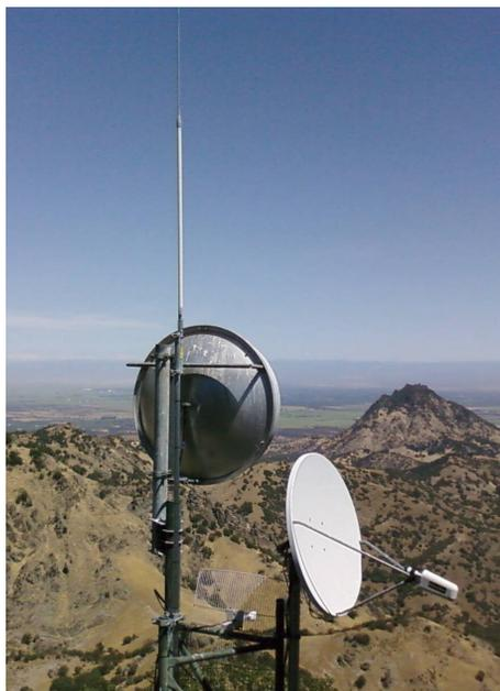
Atop the tower at 2,500' is the K6FRC/B Shakespeare PogoStick 10 meter antenna. (Courtesy: Paul Shinn K6FRC)
