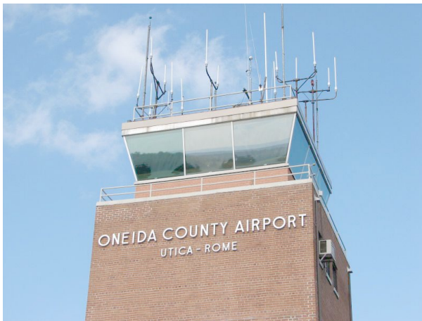
Aircraft band antennas bristle out of the top of this ATC tower in Oneida, New York. (Courtesy: Don Edwards)
