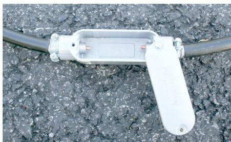
Figure 1. Loop ends secured in conduit body, cover removed.
