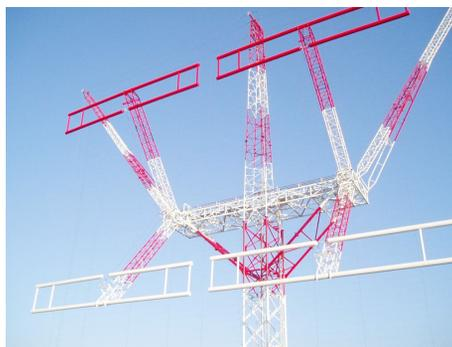
*Thomson rigid dipole antenna, a "smaller" version of the large antenna on the cover.*
