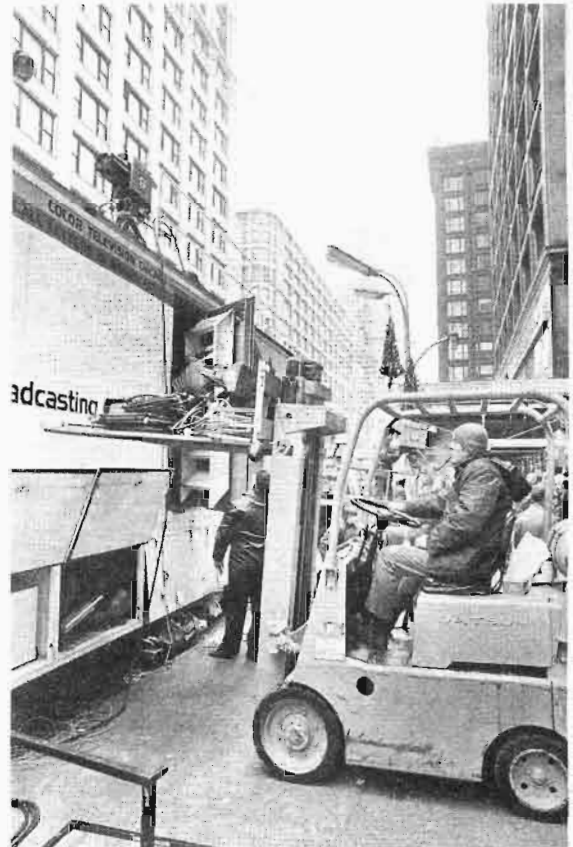
Fig. 47. Setup—raising equipment to the trailer roof.
