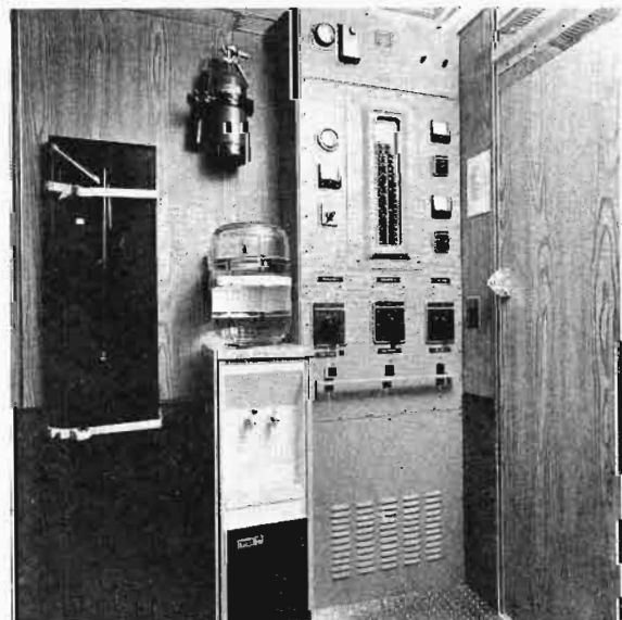
Fig. 13. Power distribution and space conditioning control.
