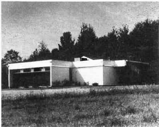
Fig. 5. View of remodeled station, WNHV in Vermont.
