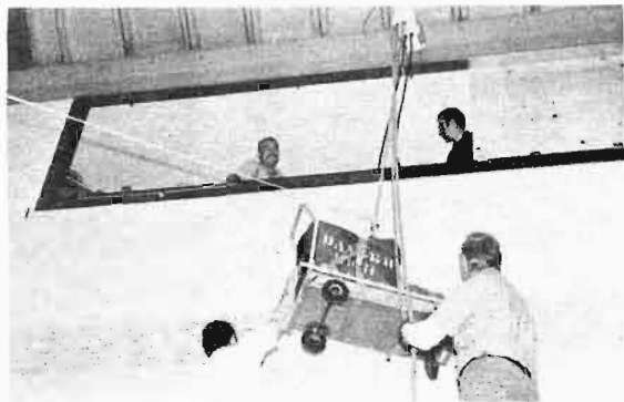
Fig. 23. Camera dolly being hoisted to football booth.
