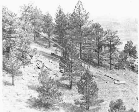
Fig. 63. Guy anchor installation at KOA-TV, Denver, Colo.
