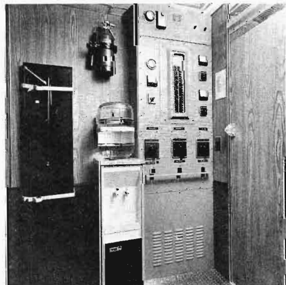
Fig. 13. Power distribution and space conditioning control.
