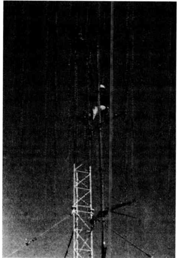
Figure 4.12-9. Three bay non-symmetrical FM antenna mounted on the tower leg. The guy cables are insulated fiber glass rods near the tower legs.
