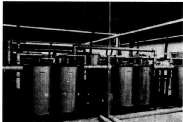
Figure 4.12-15. This Senior Road, Houston, Texas ten-port diplexing system, combines nine FM stations into one community antenna. It is capable of 350 kW total input power. (Courtesy Harris Corp.)
