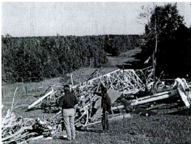
Figure 3. WLBT tower collapse, October 1997
