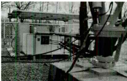
LBA ColoCoils™ in use at directional AM station with fence isolation from hot tower
