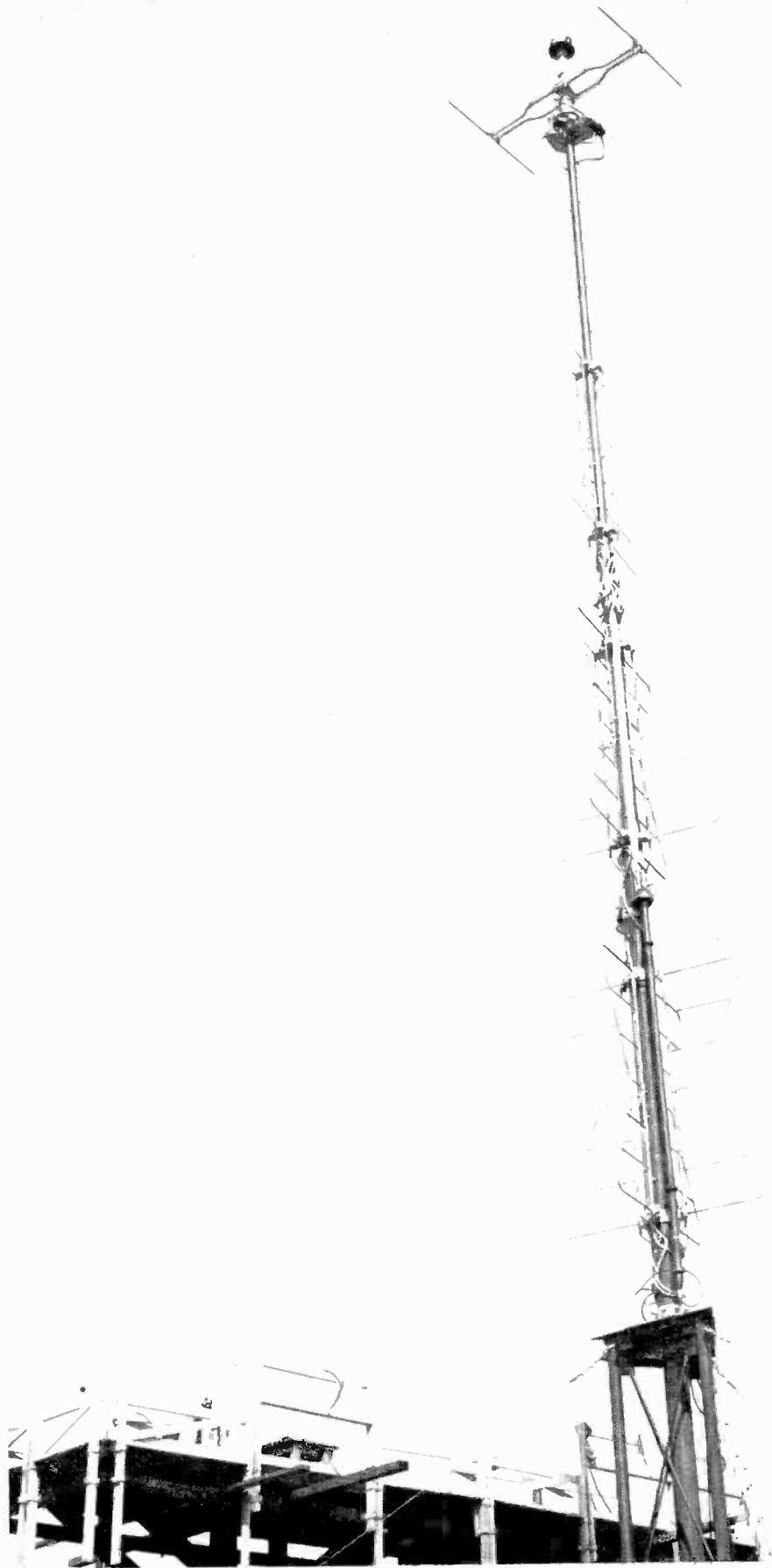
FIGURE 7 PHOTOGRAPH OF WKY-TV DIRECTIONAL ANTENNA SYSTEM SHOWING MAIN AND REFERENCE ANTENNAS
