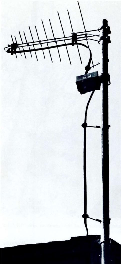
FIG. 10. New type UHF amplifiers (such as Blonder Tongue Model ABLE-U2 shown) cover entire TV spectrum.
