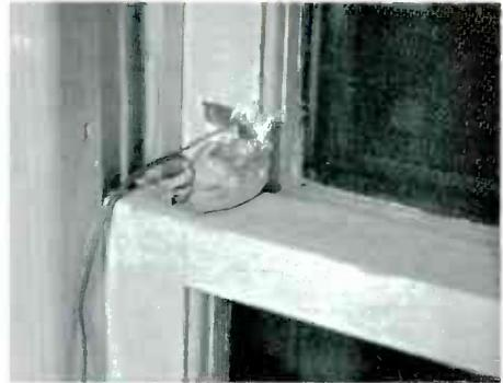
Fig. 9. (A) Microswitch installed on window; (B) Foil strip window switch.
