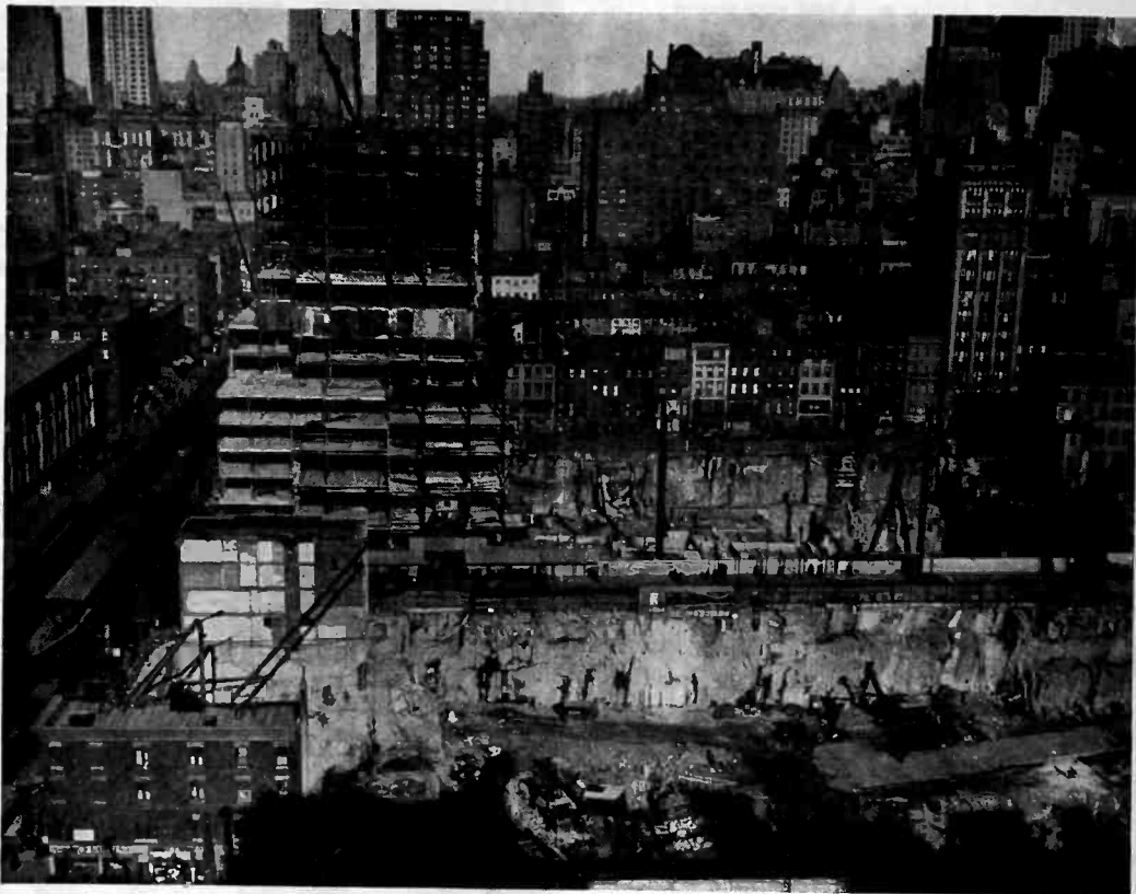
Work progressing rapidly on Radio City in the heart of Manhattan
