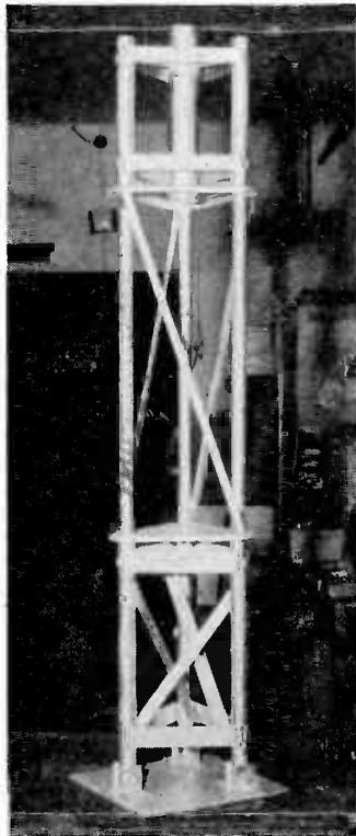
Fig. 2. One section of a typical television antenna tower. Used for heights above forty feet.
