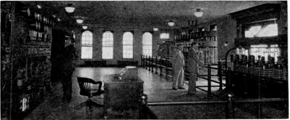
View of Main Operating Room, WENR, Chicago. Along the right wall are the high-power Radio frequency amplifiers, and the modulators, equipped with 20-kilowatt water-cooled tubes. On the left are the power supply panel, and the intermediate Radio frequency amplifier.
