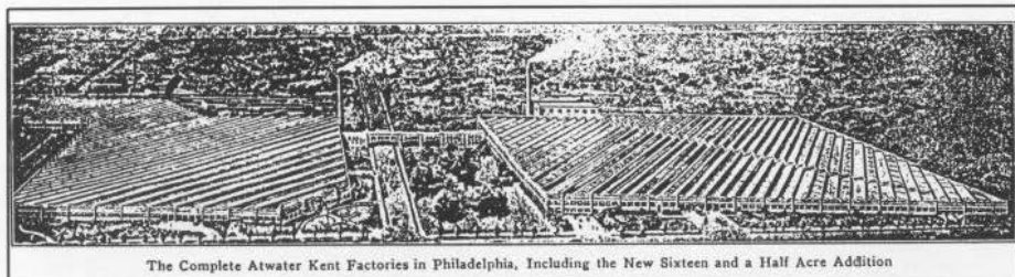
Figure 30. The 16½ acre addition to the Wissahickon Avenue plant, 1929.
