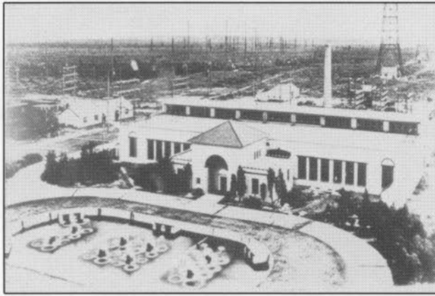
Figure 11. Another view of Radio Central in the mid-1930s. Note the poles for short-wave antennas alongside a long-wave antenna tower. The economy of short-wave antennas was one of the reasons RCA and its competitors eventually abandoned long-wave radio.
