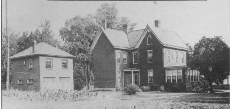
Figure 58. Conrad's garage (at left) in Wilkensburg, East Pittsburgh. (Westinghouse)
