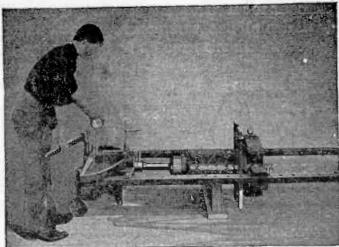
FIG. 999.—*Reliance motor construction 16.* Forcing out armature shaft.
