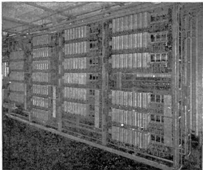
FIG. 7,663.—Step-by-step connectors mounted on switch frames.
