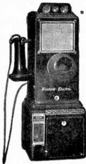
FIG. 7,525.—Coin box telephone.
