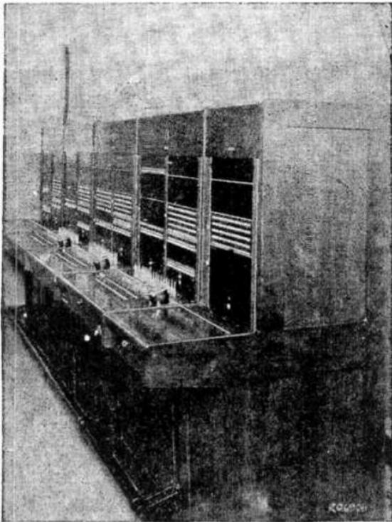
**FIG. 7,570.**—Multiple cord type P. B. X. switchboard of three positions. Note the dial on each position; this is made necessary since the P. B. X. is connected with trunk lines to a dial central office. The capacity of this switchboard without increasing the number of positions is approximately 500 lines.
