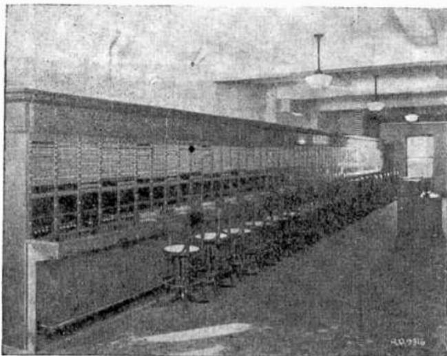
FIG. 7,571.—Large manual P. B. X switchboard.
