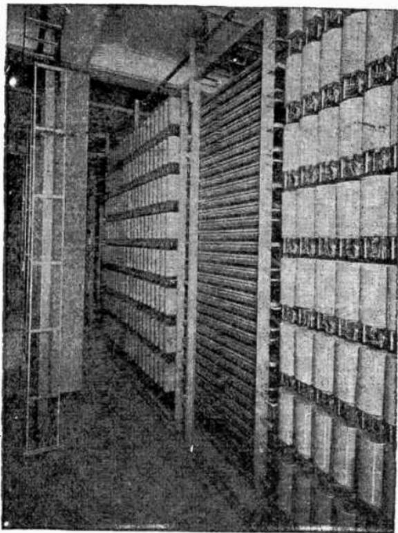
FIG. 7,674. —Groups of selectors mounted on switch frames.
