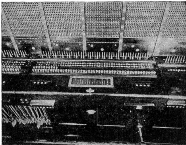
FIG. 7,566.—Typical call indicator position of a B board. The jack panels of these positions are equipped with subscriber multiple jacks like the rest of the positions on the B board. The *call indicator* box is mounted flush with the top of the keyboard.
