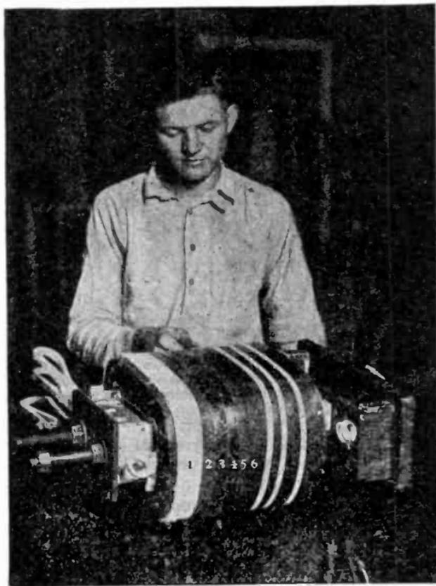
FIG. 2,313.—Wagner transformer construction 6. Coil and insulation details. 1, double cotton covered wire; 2, varnished muslin; 3, sheet mica; 4, sheet mica; 5, varnished muslin; 6, Fuller board.
