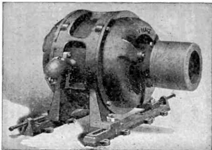
FIG. 2,555.—*Reliance induction motor construction 19.* Motor complete with slide rails and pulley.
