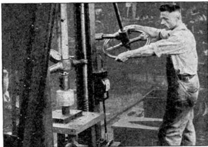
FIG. 2,542.—*Reliance induction motor construction 9.* Armature laminations are assembled under 5 tons pressure.
