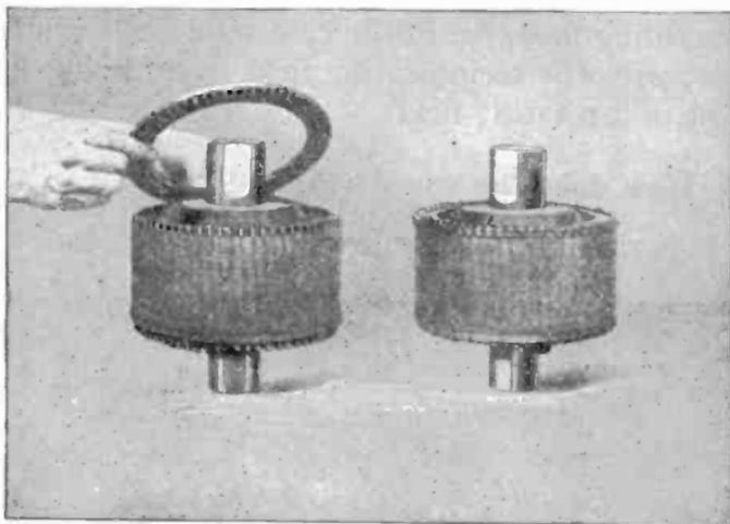
**FIGS. 2,543 and 2,544.—Reliance induction motor construction 10.** Fig. 2,543, armature with punched copper end ring ready to be placed over extension of bars; fig. 2,544, armature ready for electric welding of bars to end rings.
