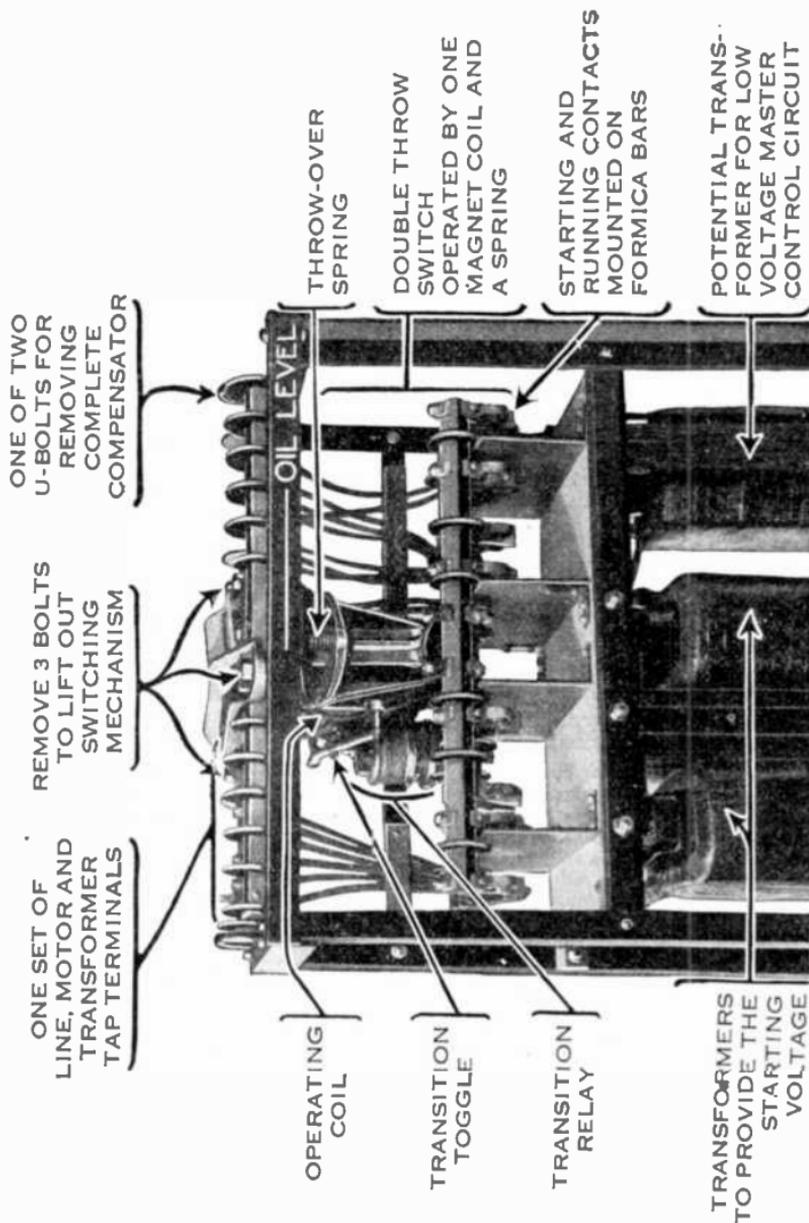
FIG. 2,693.—E. C. and M. automatic high voltage compensator removed from the oil tank to show construction. *In operation*, the double throw action of the switching mechanism is obtained by a magnet which compresses a spring when the starting contacts are engaged, and a relay which trips a knee joint toggle when the motor is up to speed, causing the starting contacts to open and the running contacts to close.
