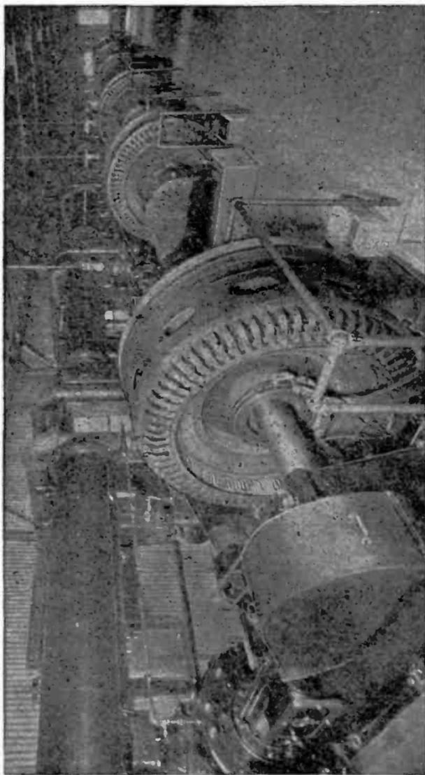
FIG. 2,506.—Six 300 *h.p.* Westinghouse synchronous motors driving air compressors furnishing compressed air for subway construction. These motors are extensively used for driving air and ammonia compressors, pulp grinders, pumps and similar applications. They are built 50 and 60 cycles, 2 and 3 phase, 100 *h.p.* at 400 *r.p.m.* to 5000 *h.p.* at 100 *r.p.m.*
