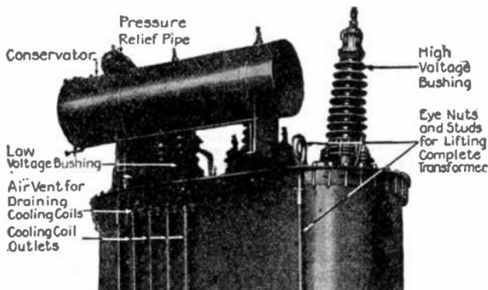
FIG. 2,369.—Top of General Electric three phase water cooled outdoor transformer with oil conservator.
