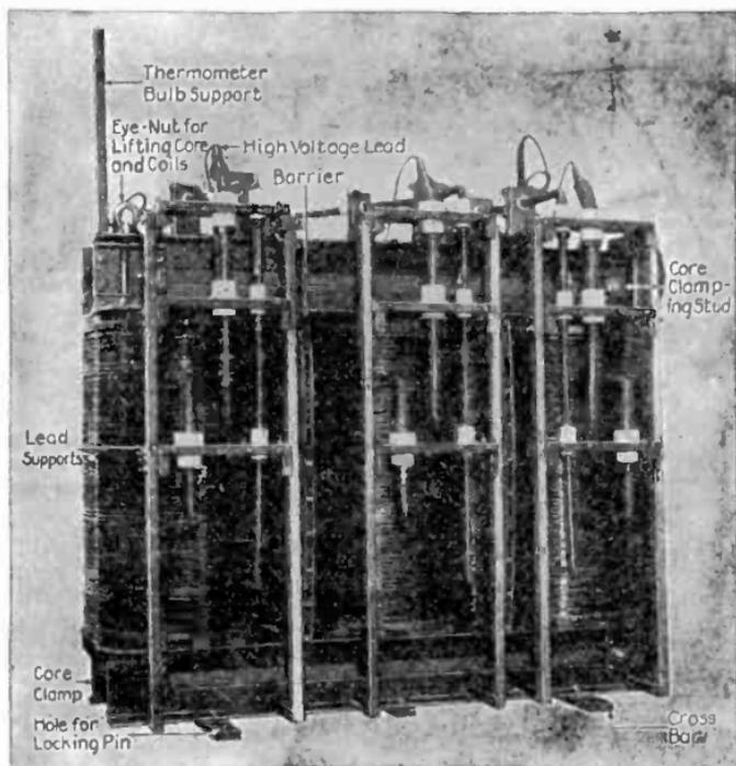
FIG. 2,364.—General Electric three phase 13,200 to 66,000 volt auto transformer. High voltage neutral solidly grounded. Interleaved disc windings.
