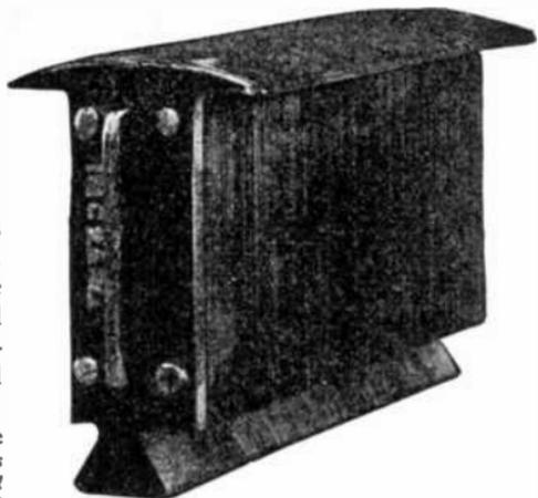
FIG. 2,269.—Wagner laminated pole piece with horns stamped in one piece. The laminations are held together between two end pieces by through rivets, as shown.
