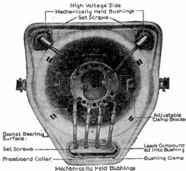
FIG. 2,373.—Top view of 2,300 volt distribution transformer showing location of core and coils in tank and method of clamping pocket bushing.
