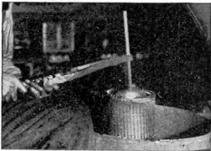
**FIG. 2,545.—Reliance induction motor construction 11.** Welding operation. Bars and end ring are welded into one solid mass to prevent loose connections.
