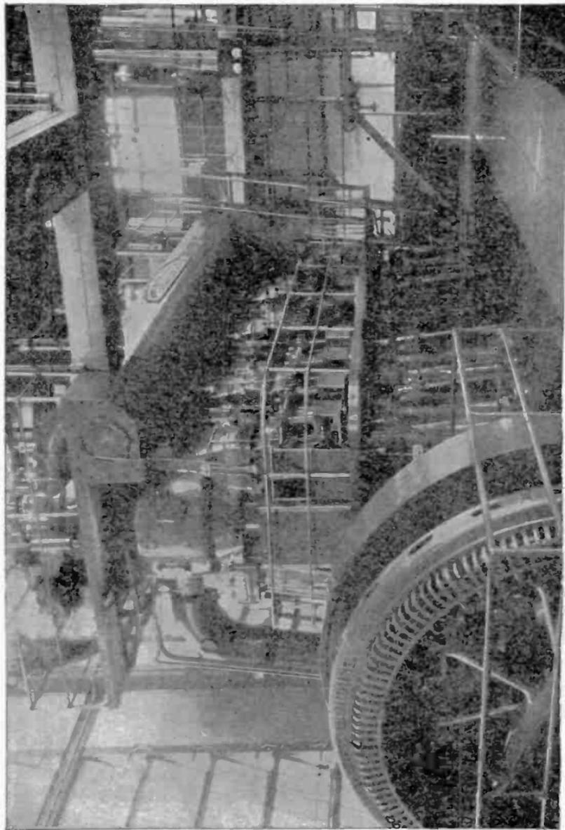
FIG. 2,186.—Westinghouse 1,600 kw. alternator direct connected to 2,250 h.p. Nordberg Diesel engine as installed in the Punta Gorda Diesel Electric Station of Florida Power and Light Co.
