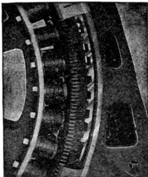
FIG. 2,285.—Section of General Electric alternator showing method of dovetailing core laminations to frame. The latter is made in two general styles, known as the *box type* and *skeleton type*. The *box type* consists of a single casting for the smaller sizes, but for large capacity alternators, the frame castings are usually divided into upper and lower sections. The *skeleton type* consists of two side castings between which substantial spacing rods are set at
