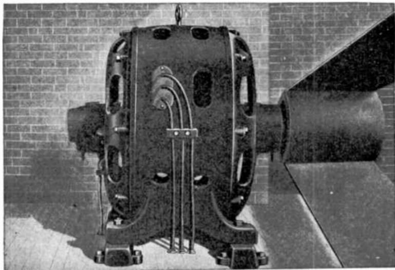
FIG. 2,221.—Allis-Chalmers high speed belted type alternator. The small pulley at the right and the angle of the belt suggest the high speed at which such alternators are run, a 50 *kva.* machine turning 1,200 revolutions per minute.
