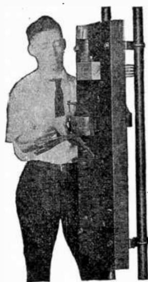
FIG. 4,185.—*How to assemble an air circuit breaker 24.* Method of placing lower stud and overload magnet frame in position on panel.
