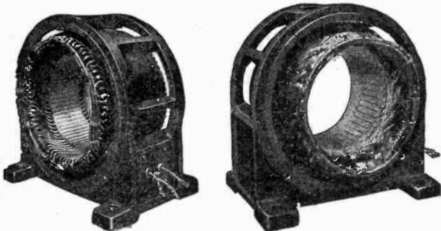
Figs. 2,798 and 2,799.—**General Electric slip ring motor construction 3.** Completed fields showing systematic arrangement of connections to facilitate reconnecting, compound insulation, batlets for leads, etc.
