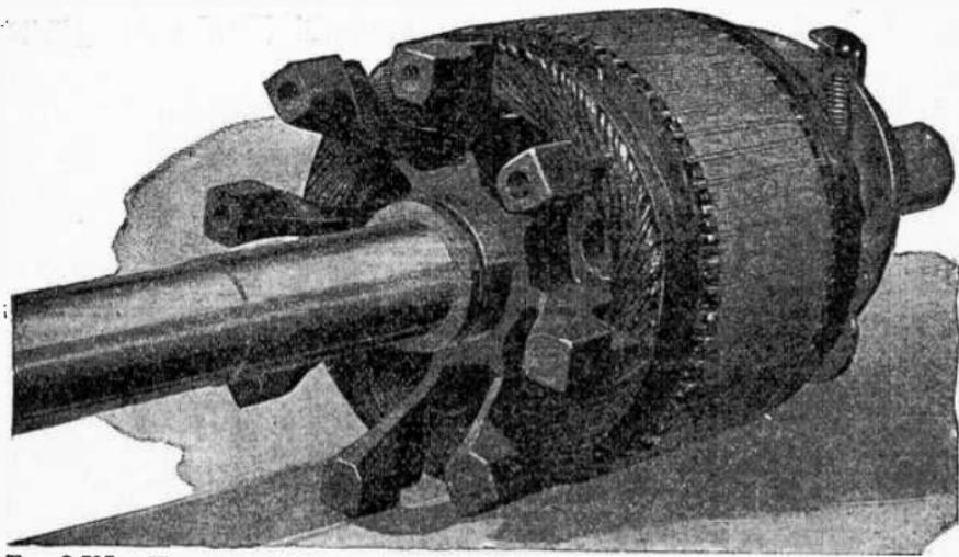
FIG. 2,707.—Wagner internal resistance motor construction 2. Another view of the armature.
