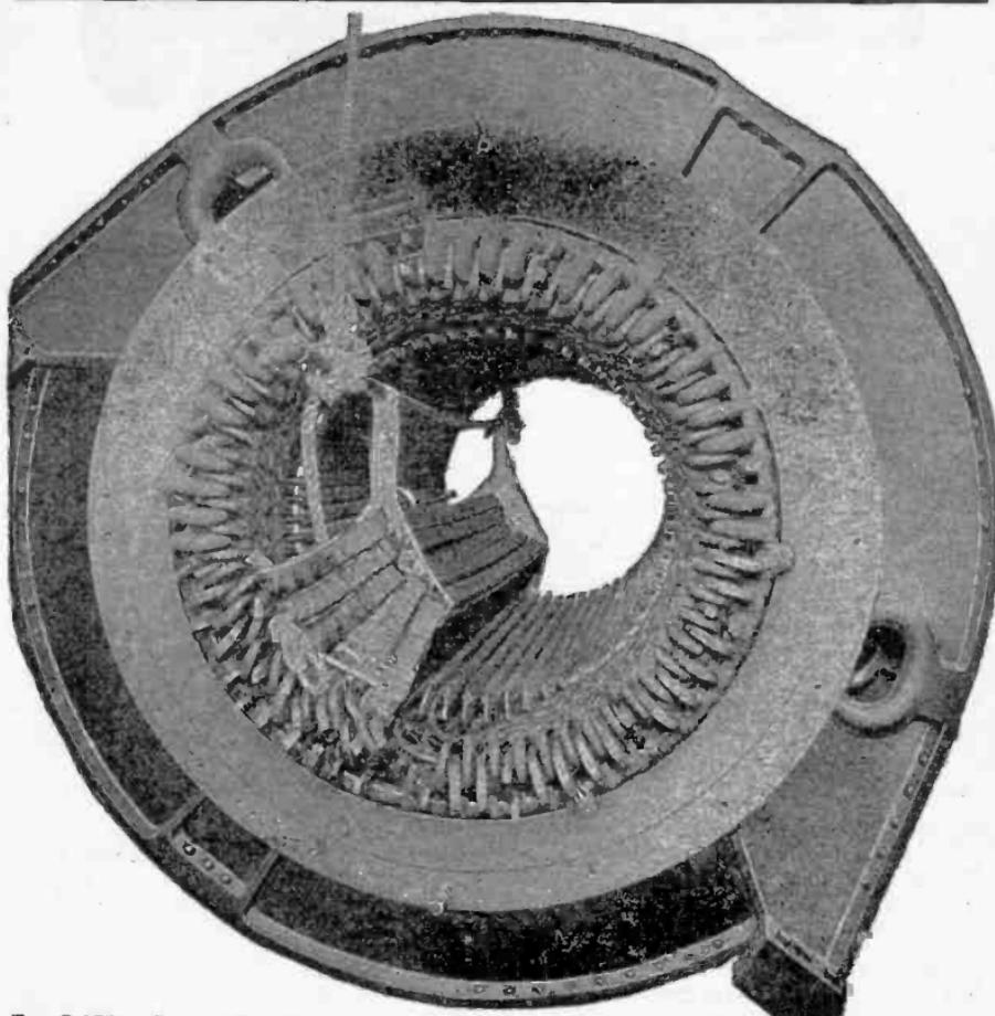
FIG. 3,155.—General Electric turbine alternator. End view showing end of armature winding and method of raising coils for inserting last coil.
