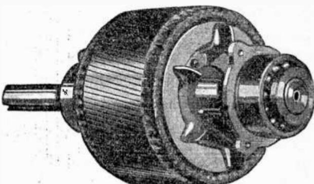
FIG. 2,768.—Fairbanks-Morse double squirrel cage armature with oblique or skewed bars.
