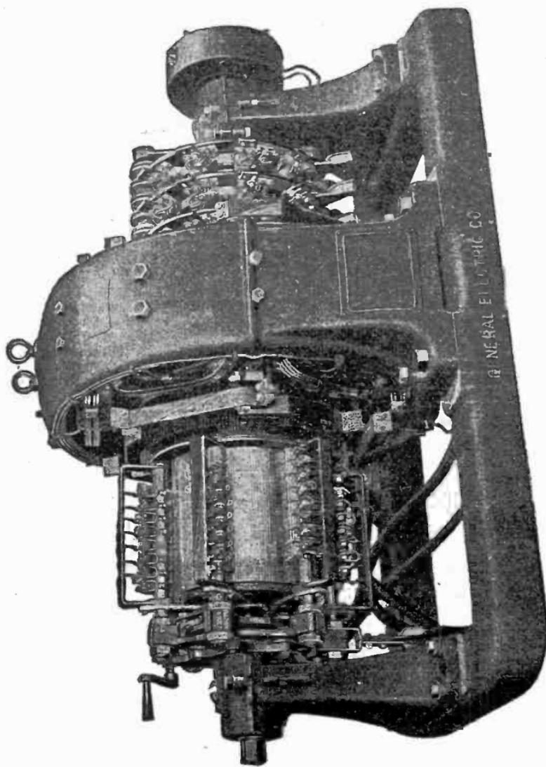
FIG. 3,088.—General Electric 300 k.w. synchronous converter for mining service. 275 volts, d.c., compound wound; 60 cycles
