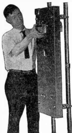
FIG. 4,184.—*How to assemble an air circuit breaker 23.* Method of placing the upper contact stud in position on panel.
