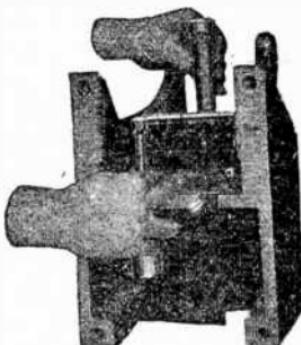
FIG. 4,144.—*How to assemble an air circuit breaker 10. Assembling closing and tripping pins.*
