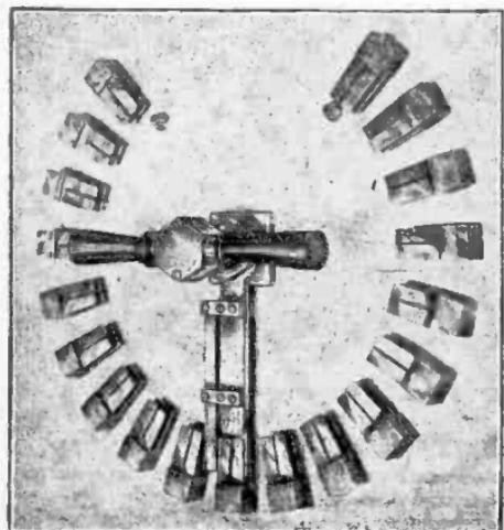
FIG. 4,052.—Metropolitan end cell switch, back connections. End cell switches are used to cut in the end cells of storage batteries as the voltage of the line drops due to discharge.
