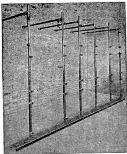
FIG. 4,634.—Pipe frame structure for a 90 inch board. The best results in a finished switchboard are obtained by first setting the frame structure accurately. Plumb and align it carefully before bolting it to the sill and wall
