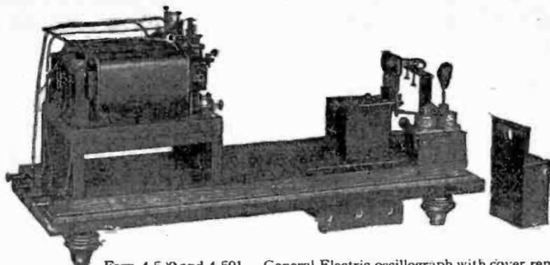
FIGS. 4,5 and 4,591.—General Electric oscillograph with cover removed.
