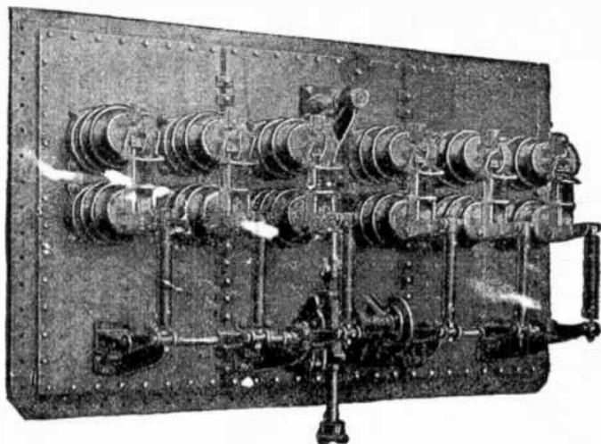
FIG. 4.511.—General Electric three phase contactor for load ratio control regulator.
