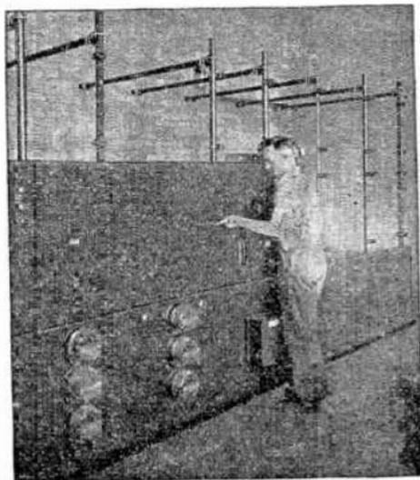
FIG. 4,635.—Erecting a switchboard of three section panels which have been shipped as individual sections. Leatheroid washers are placed between the panels and pipe fittings to align the front surface of the board. Each row of sections is leveled and aligned completely before the panel bolts are tightened.
