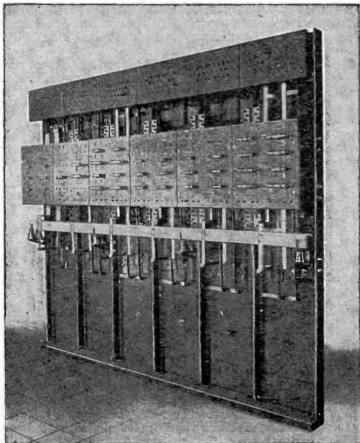
FIG. 4,724.—Rear view of Westinghouse contactor board for Keith Theatre, Boston, Mass. This view shows how the magazine panel may be mounted.
