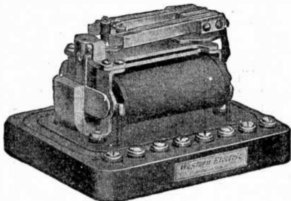
FIG. 4,800.—General Electric supervisory equipment: *Selector synchronizing relay.*
