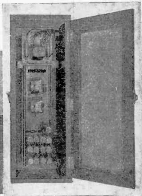
FIGS. 4,791 and 4,792.—Westinghouse audible type supervisory control apparatus; fig. 4,791 dispatcher's control equipment; fig. 4,792 sub-station relay cabinet.
