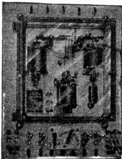
FIG. 4,326.—General Electric regulator for alternators having exciters of small capacities. When two alternators operate in parallel and the exciters are also in parallel, one regulator may be used for the control of both exciters, provided the sum of the two field currents of the two exciters does not exceed the limit for which the relay is designed. The exciters may be either shunt or compound wound.
