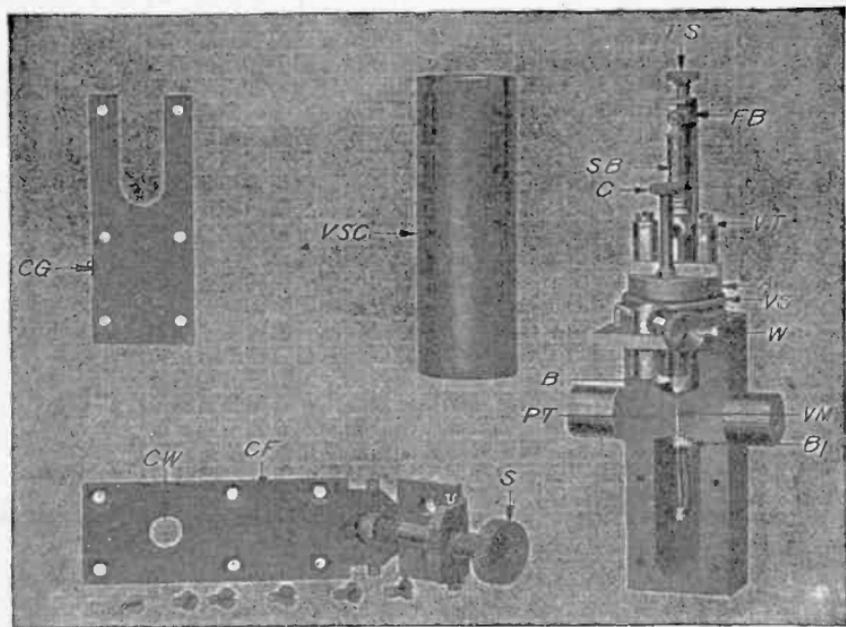
FIGS. 4,595 to 4,598.—General Electric oscillograph galvanometer cell, with front removed showing vibrator in place. *The parts are:* CG, cell gasket; VSC, vibrator shipping cart-ridge; CW, cell window; CF, cell front; PT, pole tips; VS, vibrator seat; VM, vibrator mirror; SB, spring balance; B and B<sub>1</sub>, bridges; TS, tension screw.
