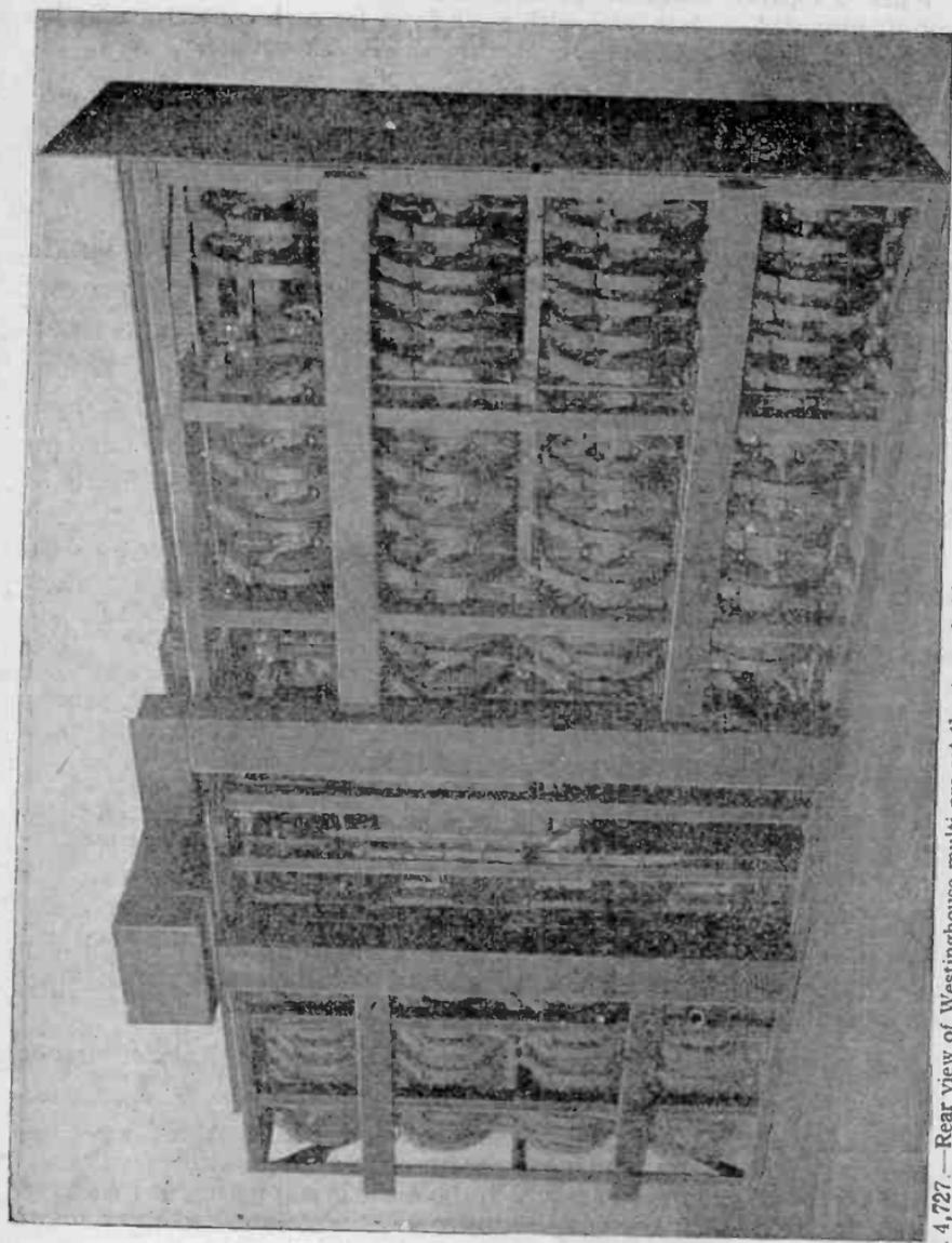
FIG. 4,727 — Rear view of Westinghouse multi-pre-set theatre switchboard, showing the mounting of the dimmers and the wiring troughs.
