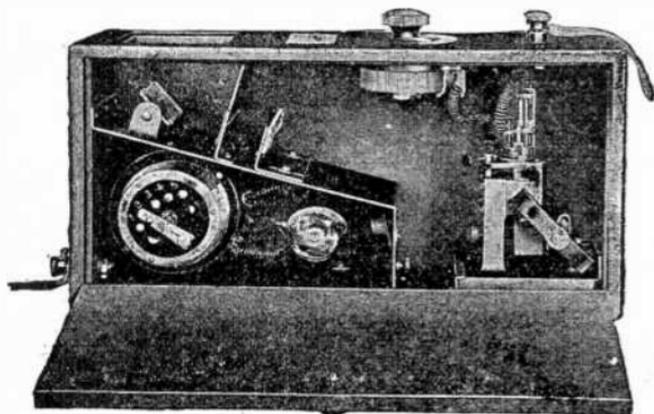
FIG. 4,623 — General Electric oscilloscope. This instrument is a simplified oscillograph having only the visual feature. *It consists of* a single element galvanometer using a high sensitivity vibrator and a permanent magnet field. A standard 6/8 volt, 21 c.p. automobile head-light lamp is the light source, a small transformer being used to adapt it for use on any 110 volt
