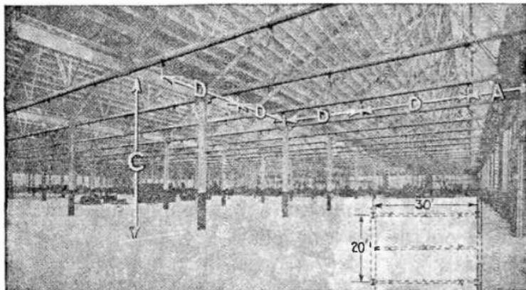
FIG. 8.403.—The layout of lighting outlets for a large industrial building. Indicating the application of data in table No. 2. The 13 foot clearance allows a spacing of 13 feet. For a symmetrical layout in the bays a 10 foot spacing is adopted.
