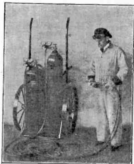
FIG. 8,147.—*Adjusting for neutral flame.* Open oxygen needle valve and adjust for neutral flame.
