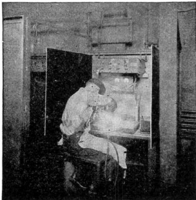
FIG. 8,071.—Position of welder when welding, showing shield, electrode, electrode lead and work table. The operator should try to assume an easy position in which the whole body is comfortable and braced so as to be steady without strain, leaving the right arm entirely free.
