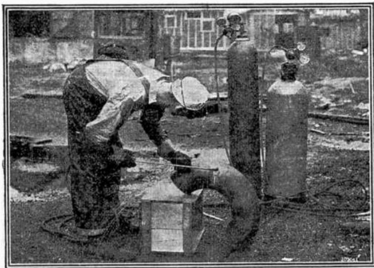
FIG. 8,187.—View showing pipe fitter cutting a 180° tube turn with oxy-acetylene torch. It will be seen from this illustration that the tube turn can be cut for a turn of any angle.
