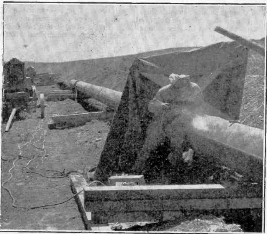
FIG. 8,170.—Section of pipe line placed on dollies on top of skids to facilitate turning of pipe during welding operations. Photographed on Uinta Pipe Line Company's 200 mile line:
