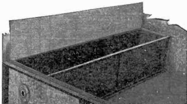
FIG. 8,744.—Buffalo suction compartment with screen cover. The settling tank is divided into two compartments by a brass wire cloth strainer, through which the water passes before entering the suction of the pump. This strainer offers a surface of more than one sq. ft. for each foot in width of the tank. The area of the strainer being many times the area of the suction pipe, provides a thorough filtering of the water at very low velocity.
