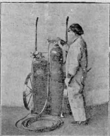
FIG. 8,140.—Connecting the hose to the regulators. (Airco-Davis-Bournonville.) Connect
