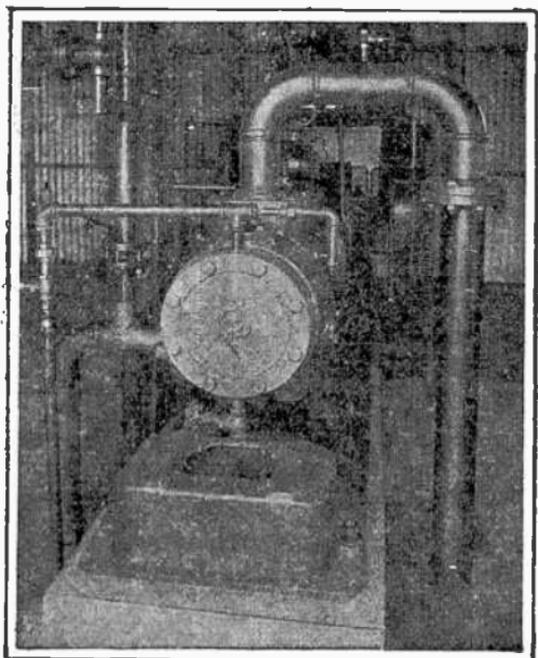
FIG. 8.188.—Gas compressor installation showing welded joint tube turn fittings in suction and discharge connections.
