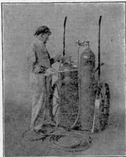
FIG. 8,144.—*Adjusting the tip.* Slip tip-nut over mixing head, screw tip into mixing head, screw tip nut into torch handle, tightening it by hand so that tip will be at proper angle.
