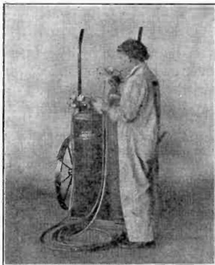
FIG. 8,142.—*Blowing out the hose.* (Airco-Davis-Bournonville.) Open each regulator with the regulator screw and blow out hose. Release regulator screws.
