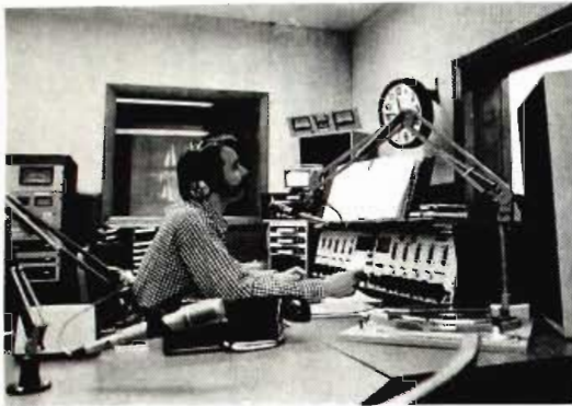
In the conversion to non-duplication, WNLK kept its stereo board in the AM (mono) control room, feeling that they could use it for additional production facilities during the station's off-air hours.
