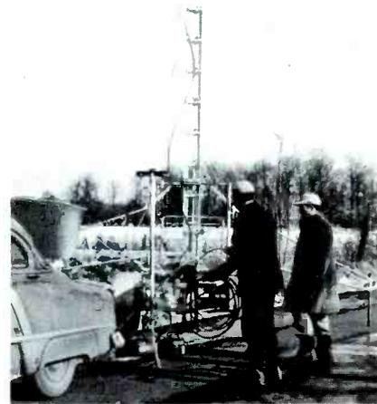
Figure 4. Installing Tubular Lead-in for Testing Purposes.
