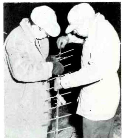
Figure 16. Photograph of the 12-Element Yagi being Prepared for Installation on the Tower.
