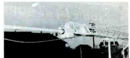
Figure 2. Insulator Standoffs Mounted on the Tower.
