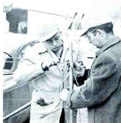
Figure 6. The Clover V-Beam (Telrex, Model 100) Being Installed on a Section of Mast.
