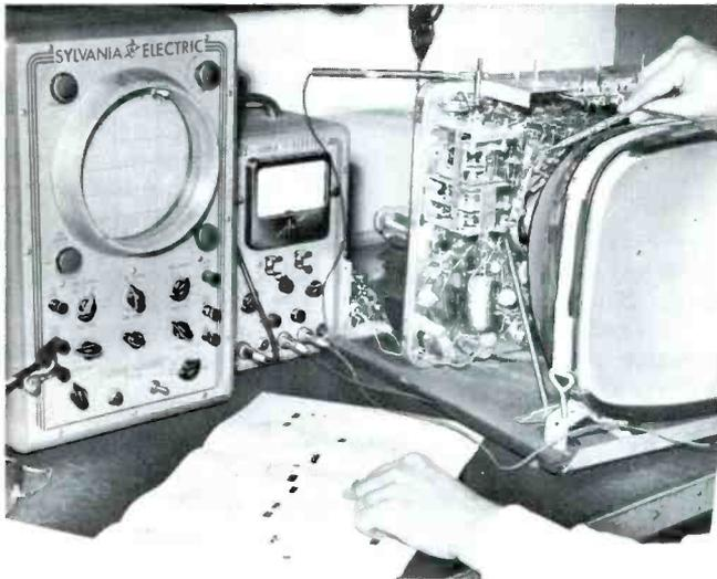
Fig. 2. Measuring Voltages on a Vertical-Chassis Receiver.
