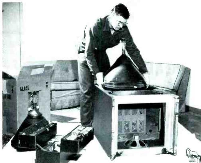
Fig. 7. Replacing a Picture Tube in the Customer's Home.
