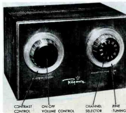
Fig. 1. Regency Model RT-700 Electronic Remote-Control Unit.
