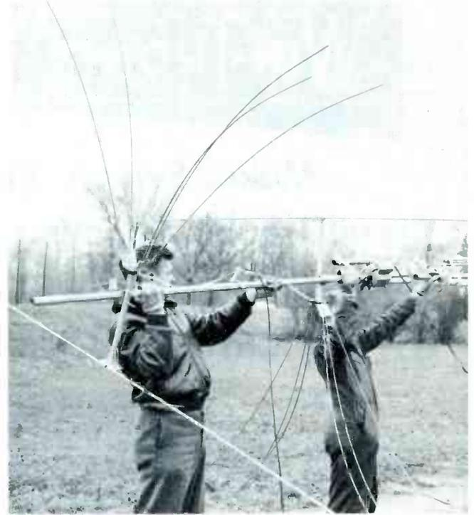
Fig. 6. Attaching Mast Assembly to Tower. ▶
