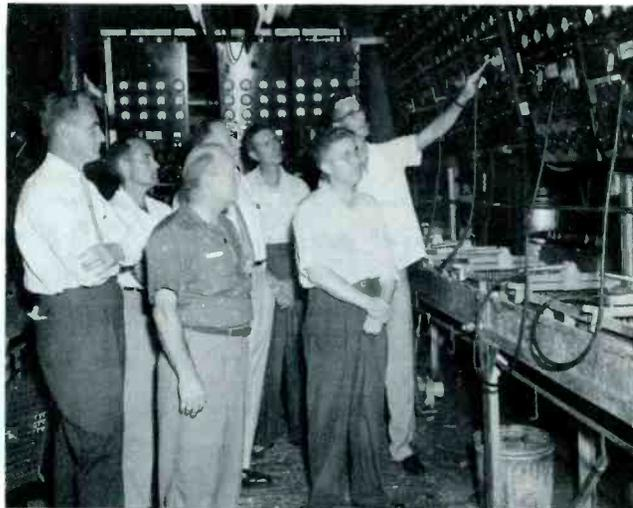
One stop on plant tour was final re-forming operation where completed capacitors are given several-hour final aging.
