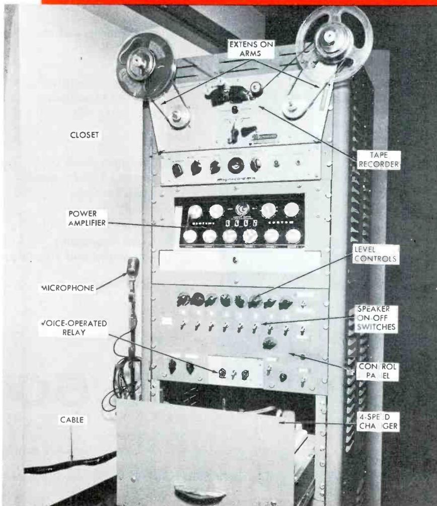
Fig. 1. A representative commercial sound installation.
