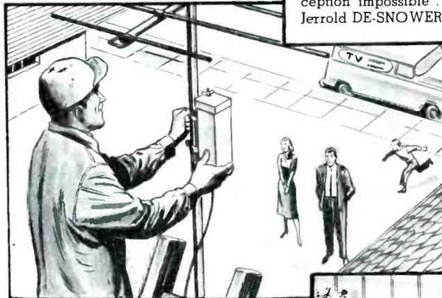
Antenna mounted, the DE-SNOWER captures the signal before loss and noise affect it, delivers it to the set over shielded coax... providing snow-free pictures.
