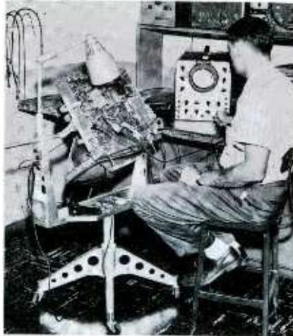
Fig. 4. Tel-A-Turn holds chassis at any desired angle for efficient servicing.
