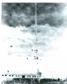
Rohn has introduced a new self-supporting communications-radio tower which can be erected to a maximum height of 170'. Formerly, the tallest tower of this type available in the line measured 130'. The increased height was gained by modifying the basic self-supporting design to incorporate three extra-heavy 20' sections. The photograph shows the new No. 170 tower installed to a height of 140'.
