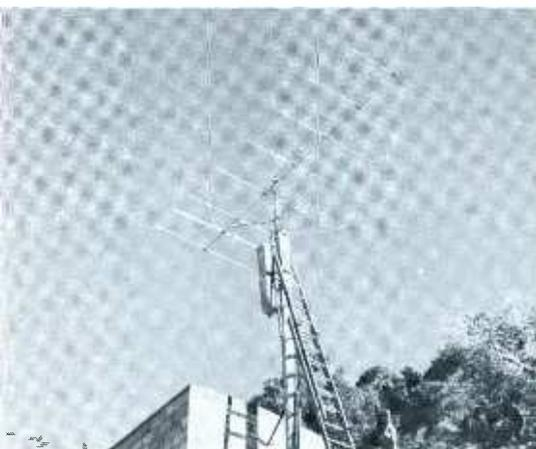
Compact installation has UHF transmitting antennas (in weatherproof housing) mounted on same mast as VHF receiving antenna. Note concrete-block shelter.
