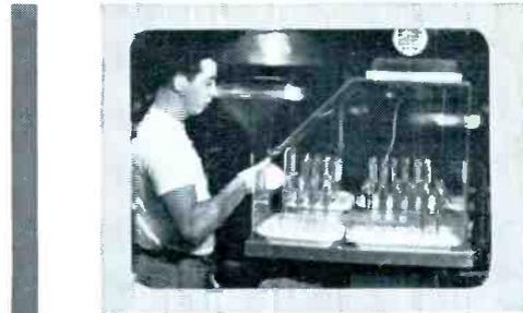
Guns await final assembly in this pressurized plastic housing. Blower at top maintains pressure, prevents dust from entering housing.
