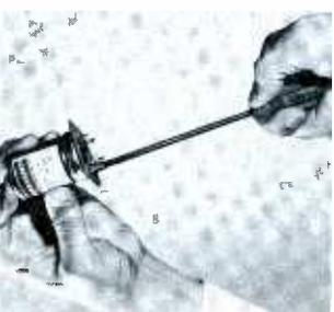
Quick twisting of tabs on electrolytic capacitors is easy with a new service aid from **General Electric**. Called a "Capacitor Tab Adjuster," the tool looks like a screwdriver, but has a slotted end instead of a blade. The slot fits over the capacitor mounting tabs, and a quick twist makes an easy job of removing and installing cantype capacitors. Price of the tool is \$1.00.
