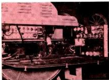
Color camera with side panels down to reveal setup and maintenance controls.
