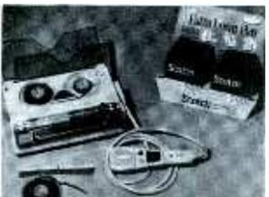
"Scotch" brand 290 is an extra-long-play magnetic tape introduced by **Minnesota Mining and Manufacturing Co.** The tape is available in 600-foot lengths on 3¼" reels. Each reel provides a full hour of recording time on two tracks at 3¾ ips. List price is \$2.95 per reel.
