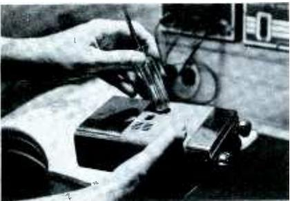
**Fig. 6. Tapping case aggravates fault.**
