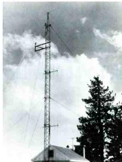
Fig. 4. Guy wires are of extreme importance on this remote relay station.
