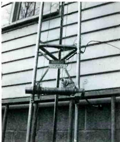
Fig. 3. Example of a crank-down tower.
