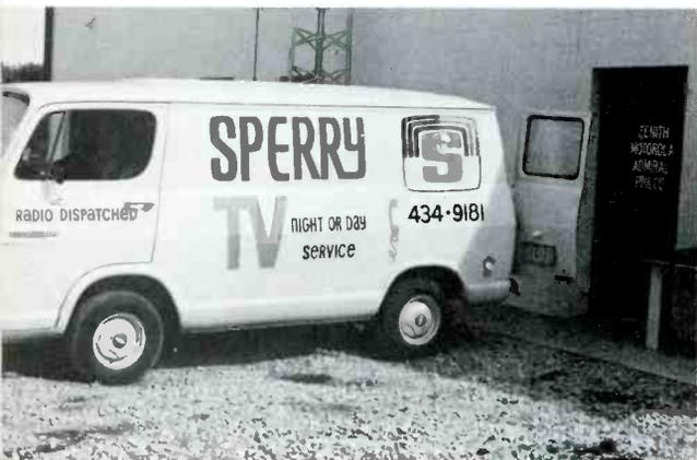
**Specialization by brand** makes technicians more efficient, and permits storage of frequently used parts close to work bench. Specialization is indicated even at back door. Outside men back the trucks up to the door that marks the entrance to the repair line for the models they are bringing in. There are four lines for major models; one for all other brands.
