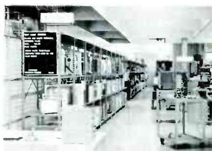
**The "air test" is made,** on the average, for a couple of days. The sets are placed here after they are repaired and double-checked. (Prices posted on the front of this rack are for "demand" customers, and do not apply to customers covered by warranty or Central's service contracts.)
