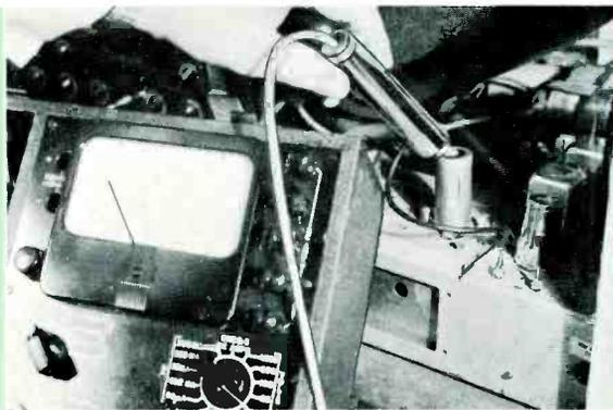
**Fig. 11** Checking local-oscillator operation.
