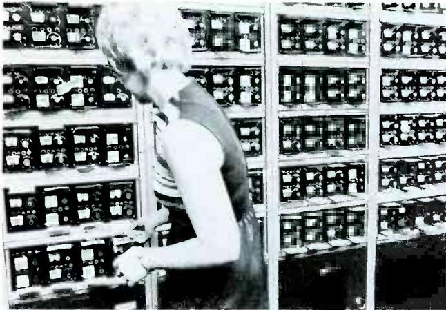
Fig. 1 Banks of monitor terminals connect by leased phone lines to fire and intrusion alarm systems located at customers' premises. Only professional alarm companies offer services like this.
