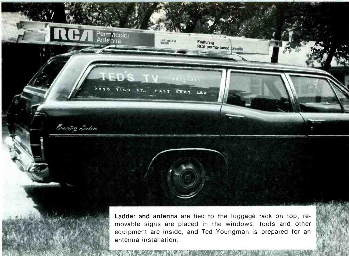
Ladder and antenna are tied to the luggage rack on top, removable signs are placed in the windows, tools and other equipment are inside, and Ted Youngman is prepared for an antenna installation.
