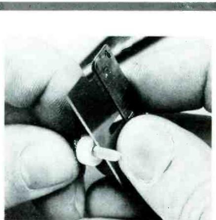
**Step 7** Gently, with the sharp blade next to the spacer, circle the insulation of the center conductor. Your object is to sever the insulation there without nicking the wire inside. If you do accidentally nick the wire, cut off the whole cable end and start all over. A nick here virtually assures you of a bad connection. The center wire will break off inside the connector—very soon, if not immediately.
