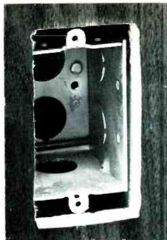
**Fig. 3** This steel outlet box has been roughed in, and is ready for the cable and tap. Large 16-penny nails go through the box and into the wood stud for a strong mounting. The knock-outs have been removed to make the cable installation easy.
