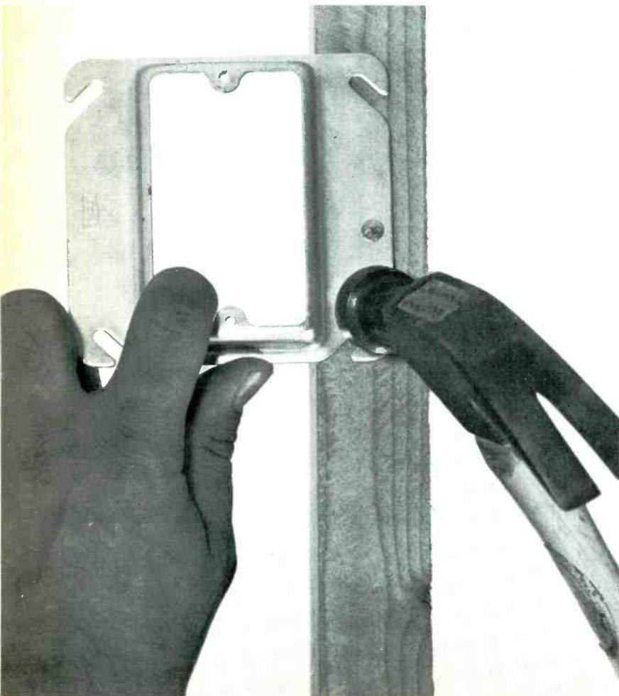
MATV system installations require more wall taps than any other kind of component. Of course, each tap must be attached to a wall, or held in position by some means. Usually the mounting devices are: electrical switch or outlet boxes; "plaster rings", plaster straps; or surface-mount boxes. Many of these are the same as the ones used by electricians for duplex outlets. Also, the locations of the wall taps are similar to where AC outlets are placed.
